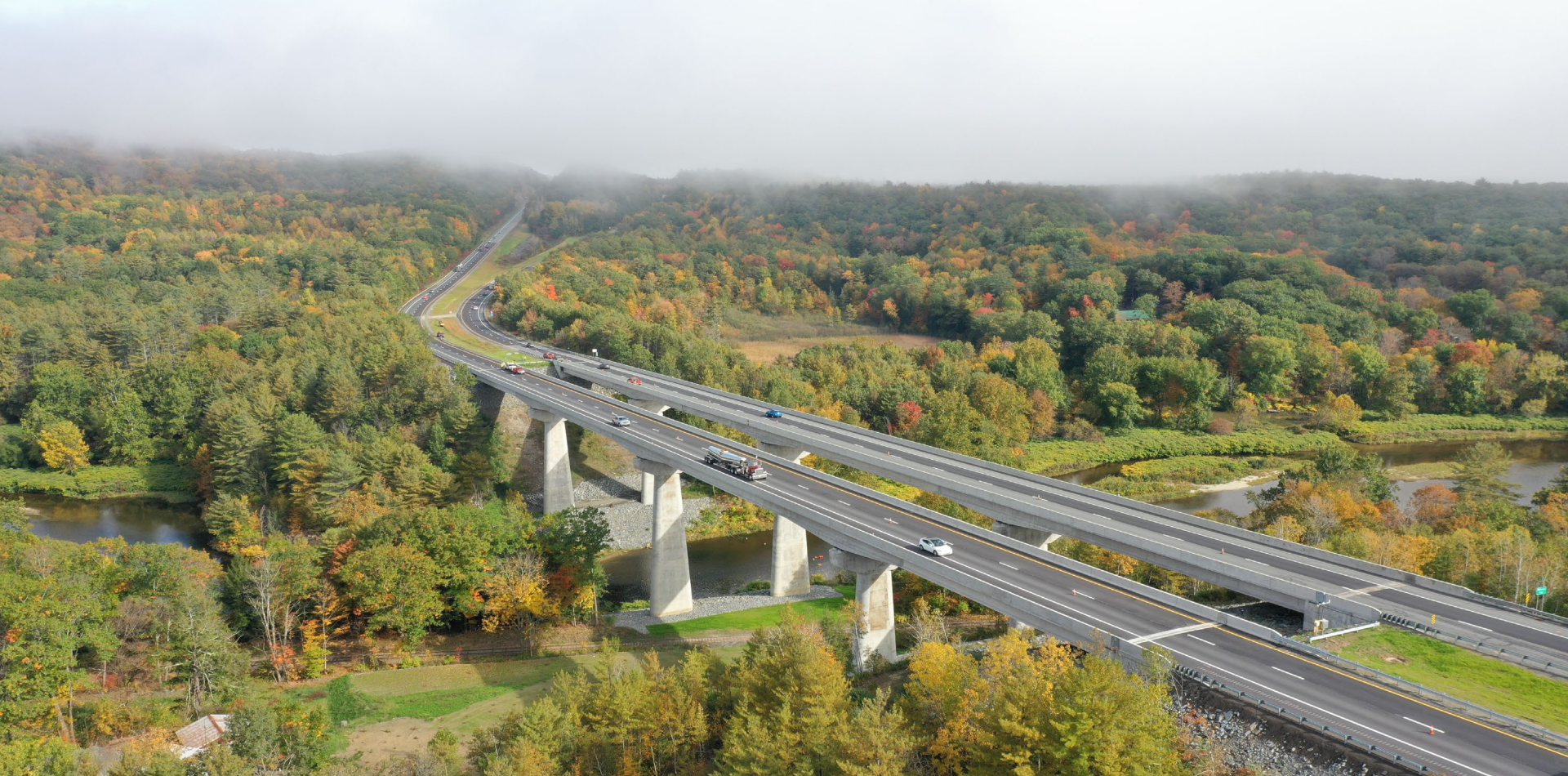
(Drone Picture of Completed Bridge – October 2021)
